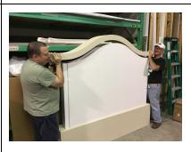
6. Run a bead of silicone adhesive (included) on top of each sign board edge and carefully place the cap onto the sign face. Be careful not to use too much adhesive and clean up any excess. Then have two people lift cap over sign face. The cap may or may not be a tight fit depending on the version you have. Align it properly on the sign face.
