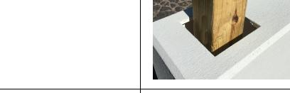
2. The height of your wood posts that are sticking out of the ground is determined by the overall height of your assembled sign components (minus 4").
