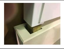
4. Then pick up the main sign section and slide over the wood 4x4's. This main sign section will rest on top of the pedestal base top as shown in step #5.
