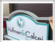
5A. Run a bead of construction adhesive (included) on top of sign board edges and place cap onto sign face. Be careful not to use too much adhesive and clean up any excess. Slide the sign cap back and forth and side to side to align it properly.
