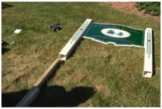
5. Lay sign down and slide treated wood posts (or aluminum I beams) up into bottom of sign posts. (If using Aluminum I beams the flat side of the beam will be facing up in this step. So the "opening" on the side of the I beam will face inward, allowing room for your sign "tabs" on either side.)
