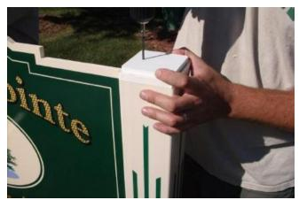
4. Screw top of clip down to top of sign "tab" on inside of posts.
