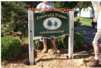
8. Pick up entire sign and carefully lower into holes. Check for level and straighten accordingly. For our very large signs, you may choose to add "post-hole" concrete to your holes prior to backfilling with the dirt. ("Post Hole concrete" does not need to be premixed, you can just pour into your hole straight from the bag and then pour water on top of it, it will harden up on its own then.)
